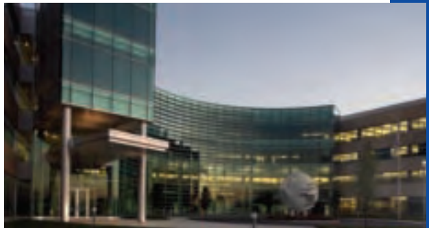
Located in the heart of Milwaukee County's Research Park in Wauwatosa, GE Healthcare's newest Southeastern Wisconsin facility is home to more than 2,000 employees.
